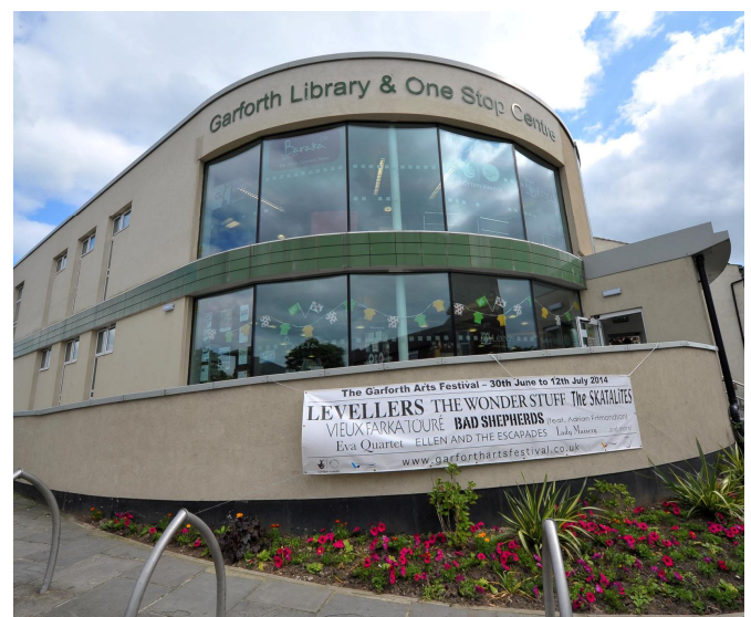
Garforth Library and One Stop Centre on Main Street
